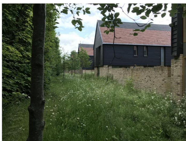
Figure 48. Good quality boundary treatments, including to rear and side boundaries, are durable, attractive and complement the landscape setting. Example: Great Knighton, Cambridge.
