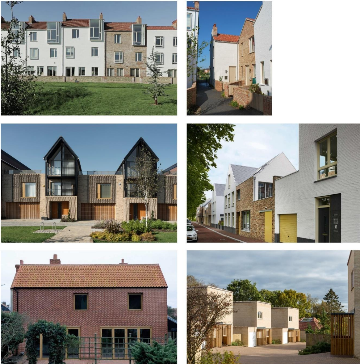
Figure 19. New housing developments creating attractive places at a range of scales that successfully address the public realm and use materials relevant to the Great Yarmouth context.
