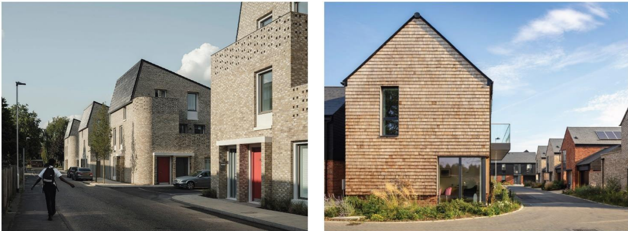
Figure 39. Good design creates successful enclosure of streets and public spaces, and ensures corners are turned without blank flank walls.
